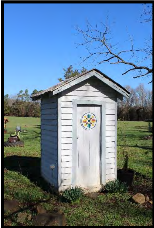
Figure 14: Moser Farm, Shed, Looking North.
