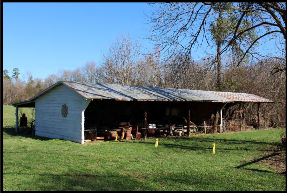
Figure 16: Moser Farm, Stable, Looking North.
