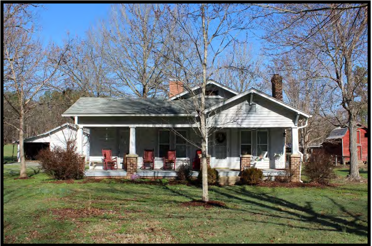
Figure 3: Moser Farm, Looking Northwest.
