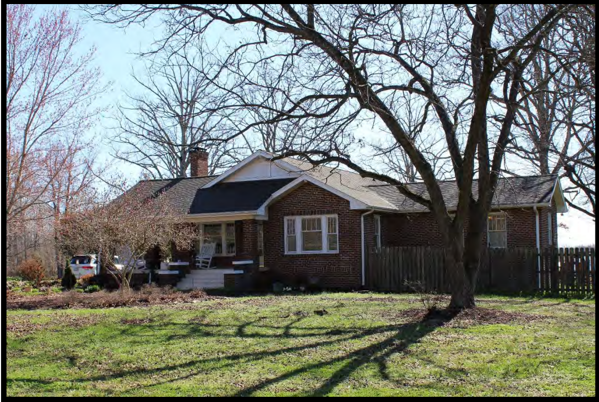
Figure 24: 3016 NC 62, Looking East.
