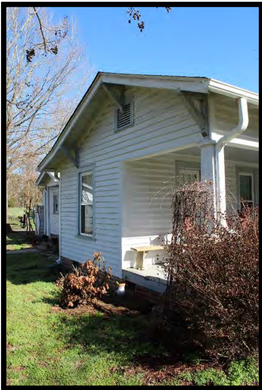
Figure 5: Moser Farm, Typical Gable.
