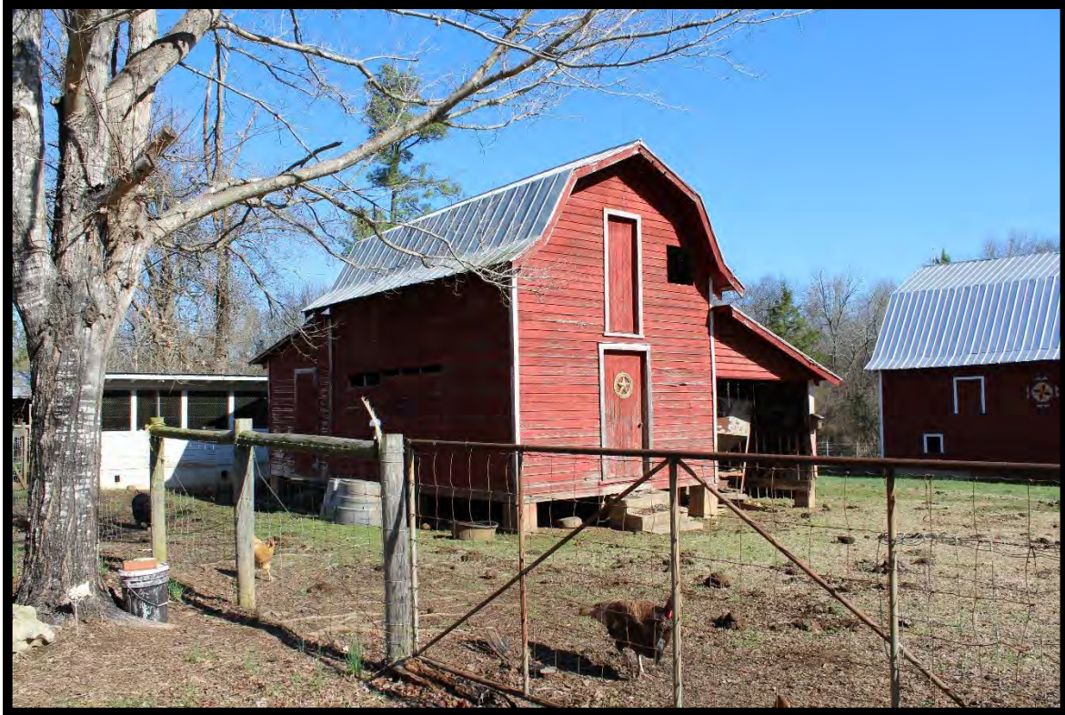
Figure 18: Moser Farm, Small Barn, Looking North.
