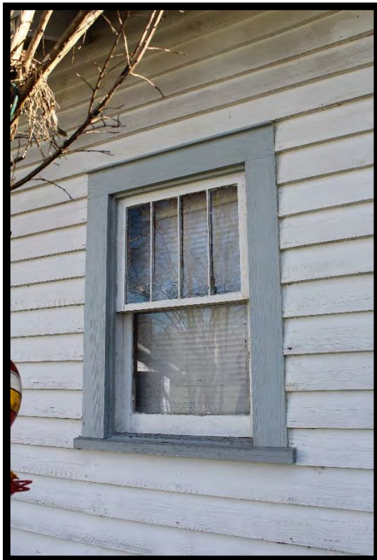
Figure 9: Moser Farm, Original Wooden Sash Window.
