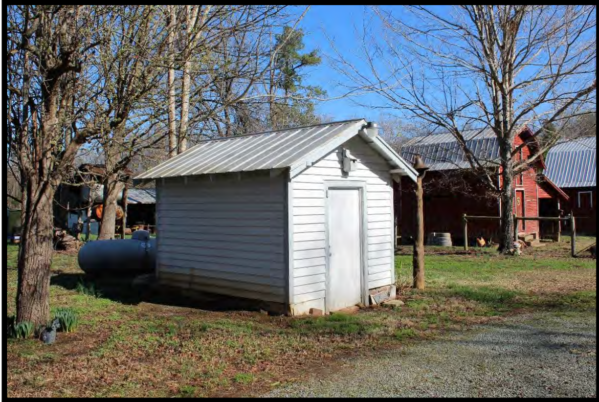
Figure 13: Moser Farm, Shed, Looking North.
